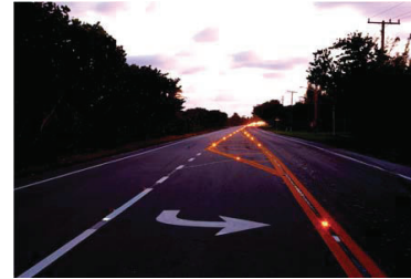
SR A1A, Boca Raton, Florida: Internally illuminated LED pavement markers provide delineation at night when pole mounted lights are turned off during sea turtle nesting season (Photo by Erdman Anthony & Associates, Inc.).
